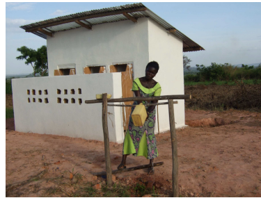
Type of latrine built by IPASC for community use
